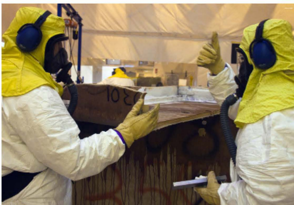
Crews repackage waste to be shipped to the Waste Isolation Pilot Plant.
